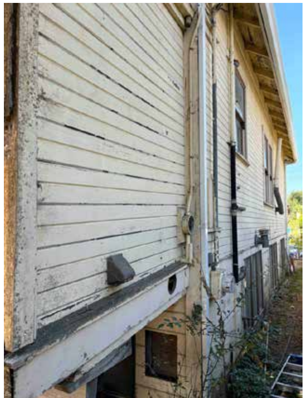
Fig.11 - 60 Third St. – Northeast side, from rear
