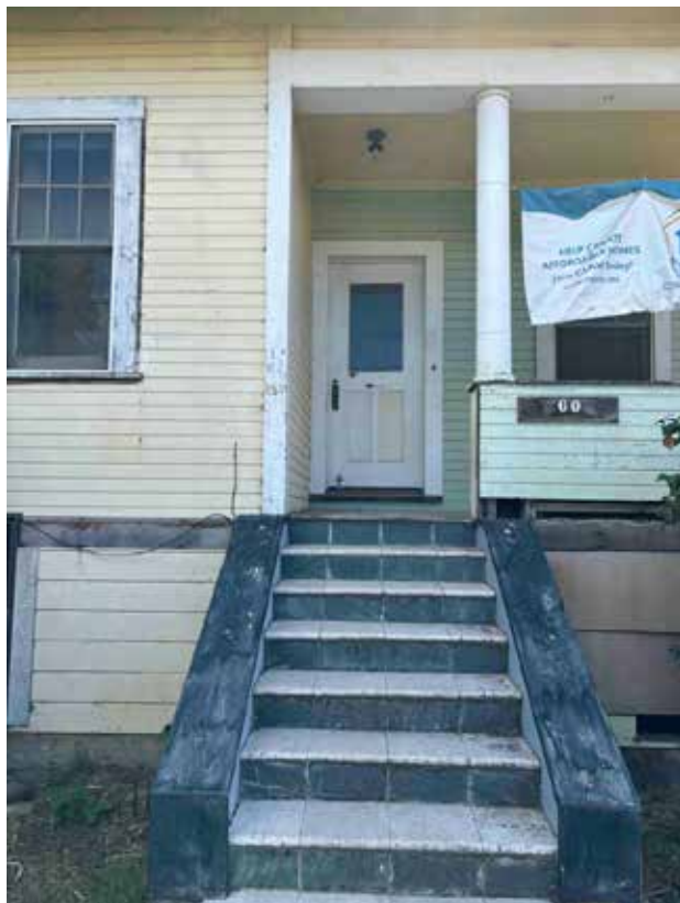
Fig.10 - 60 Third St. – Front entry and porch
