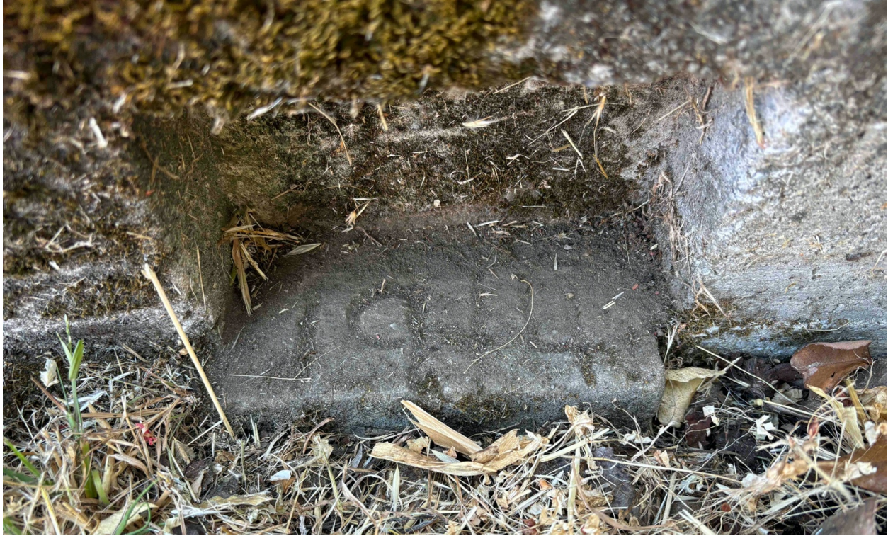
Fig.5 - 60 Third St. – Inscribed concrete at base of entry stair
