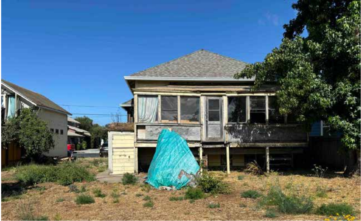
Fig.12 - 60 Third St. – Rear (southeast)
