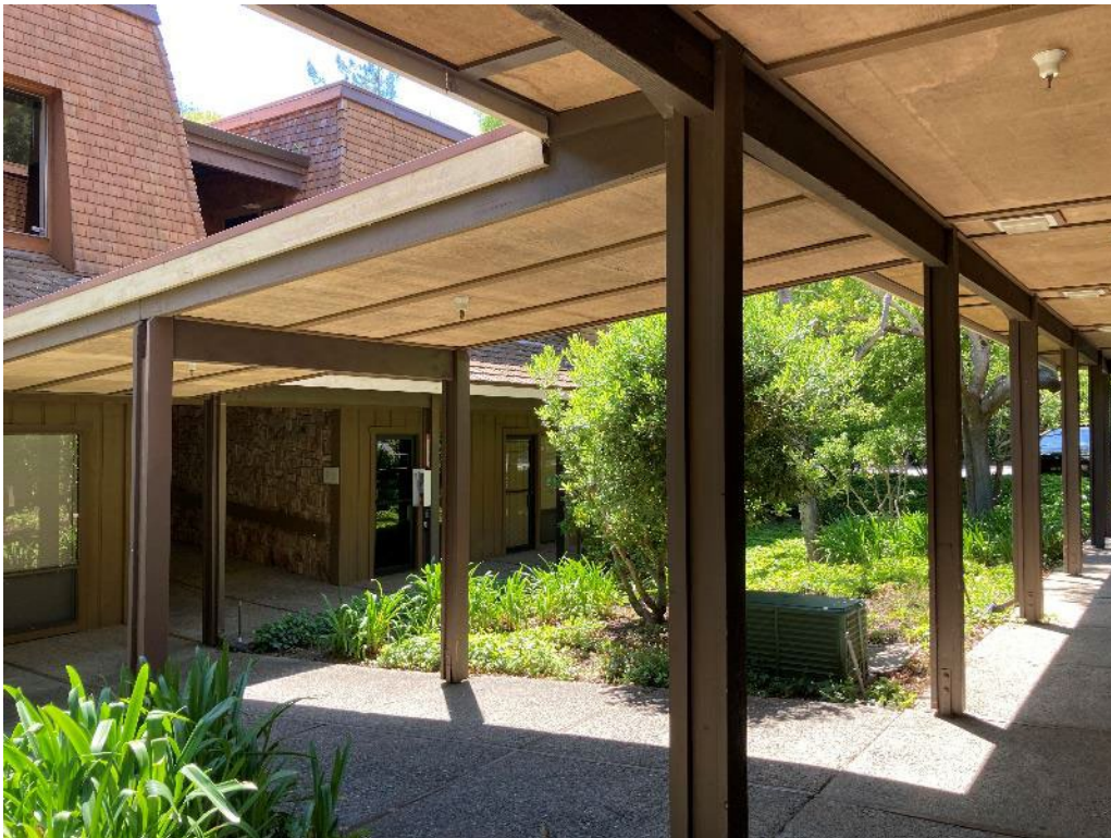
Photo 2. Covered breezeway. Ascent 2024.
