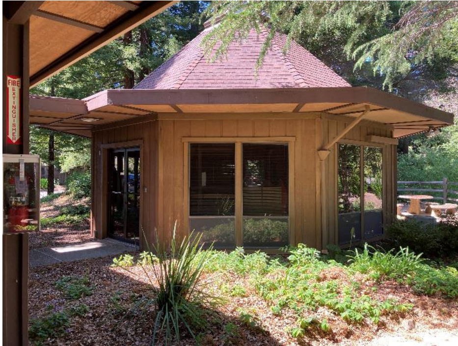
Photo 3. Semi-detached conference room, breezeway roof attached to northernmost office building. Ascent 2024.
