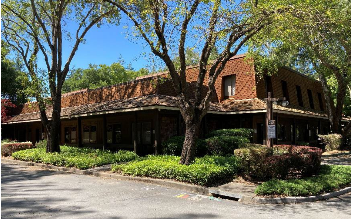
Photo 5. South façade of southernmost building. Ascent 2024.
