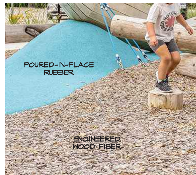
ACCESSIBLE SAFETY PLAY SURFACING
