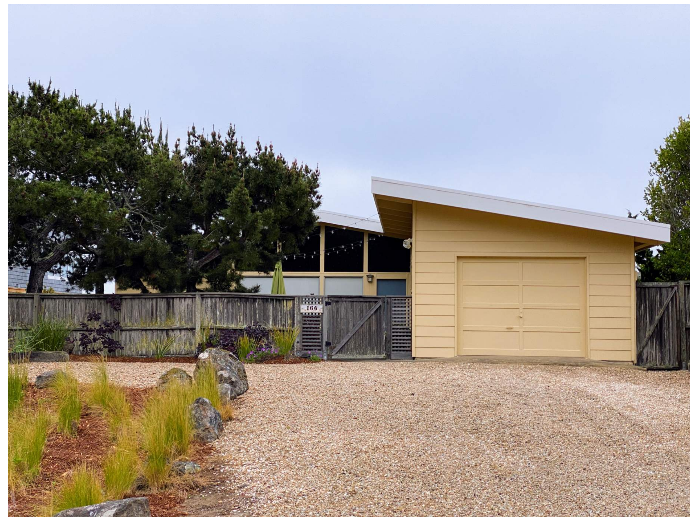
EXISTING HOUSE FROM DRIVEWAY
