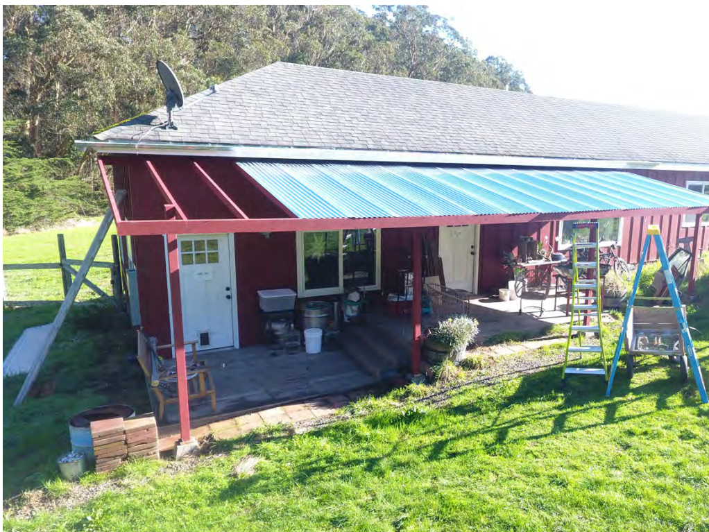
West side view
