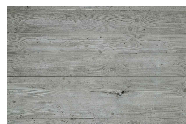
BOARD FORMED CONCRETE
