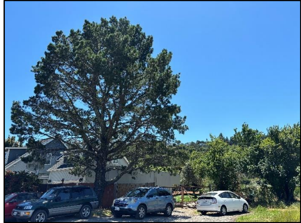
Photo 13: Monterey pine ( Pinus radiata ) had low vigor, moderate dieback and was in poor condition.
