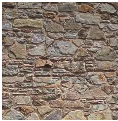
ST-01 STONE CLAD WOOD STUD FRAMED WALLS NON COMBUSTIBLE
