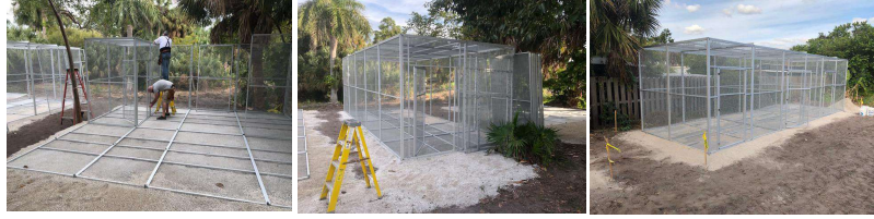
SAMPLE IMAGE: PREFABRICATED CAGING ON GRAVEL
