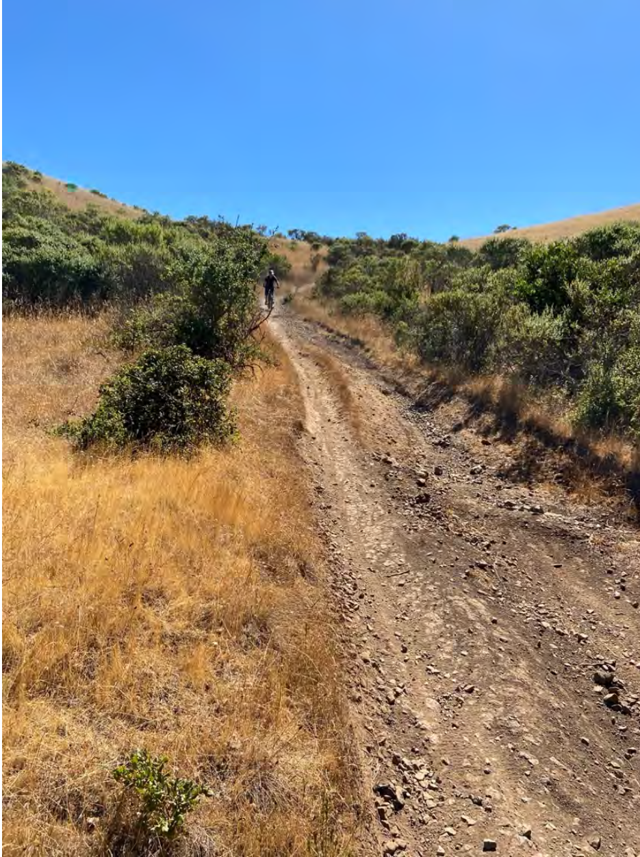
Photo 4: View of the existing Saddlecut Fire Road section proposed for restoration
