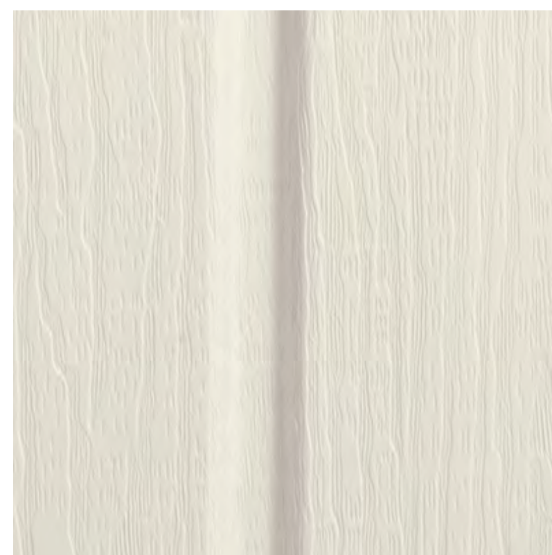
PAINTED FIBERCEMENT BOARD AND BATT SIDING ON UPPER LIGHT MONITOR WALL
