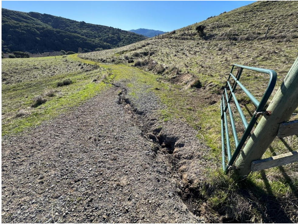
Site Photograph 13 – Looking along proposed access / utility easement
