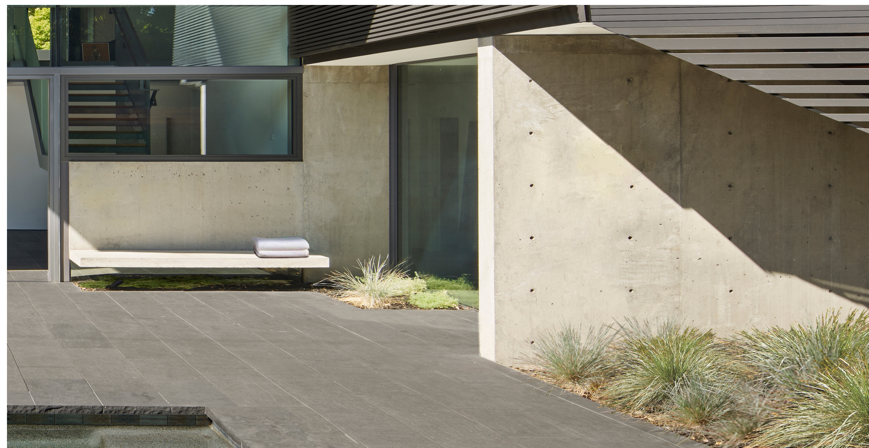
Finish Concrete - Cast-in-place MDO formed concrete. Black Basalt Stone Pavers - For decks, patios and pathways.
