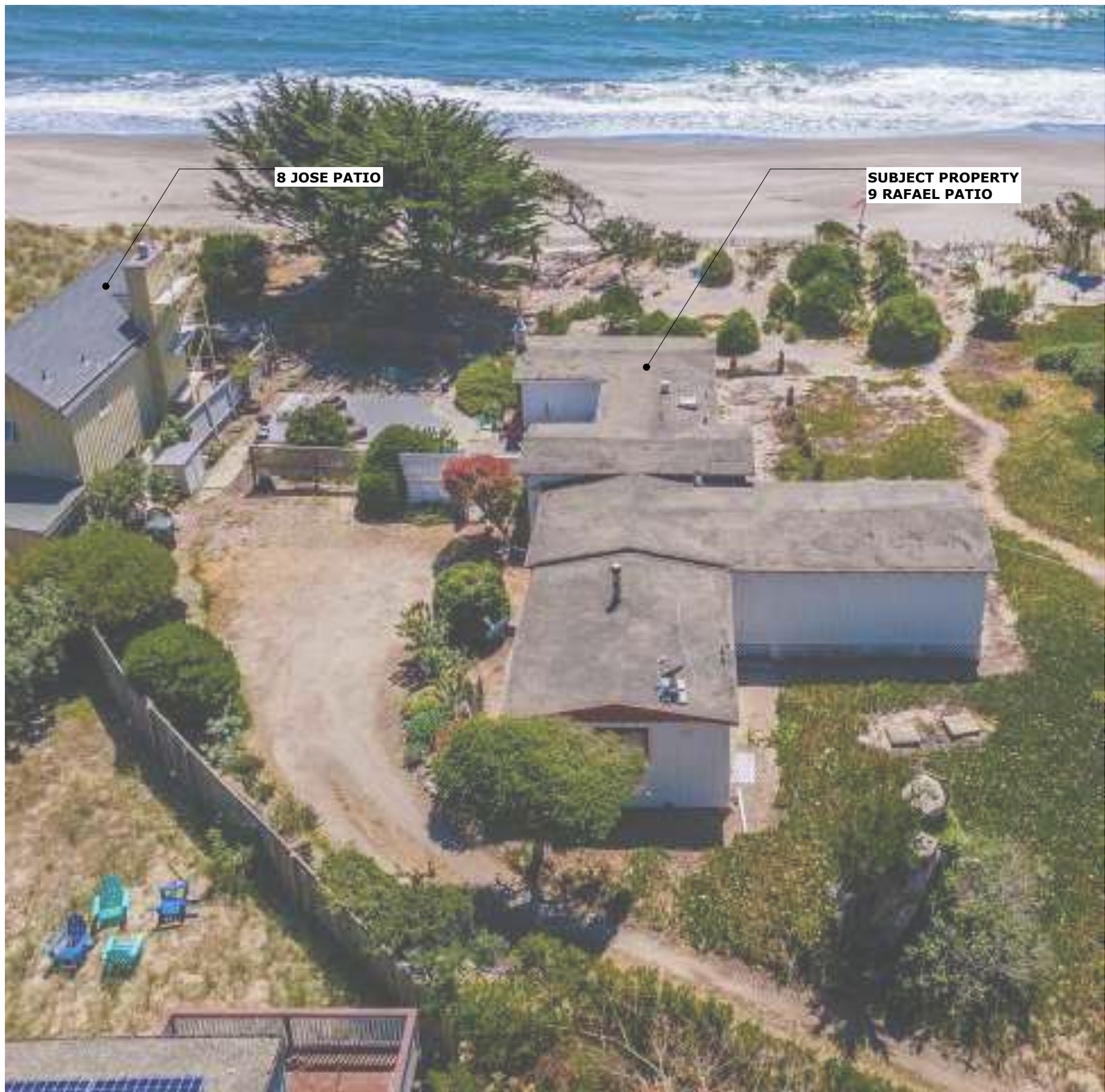
6 AERIAL VIEW SOUTH
