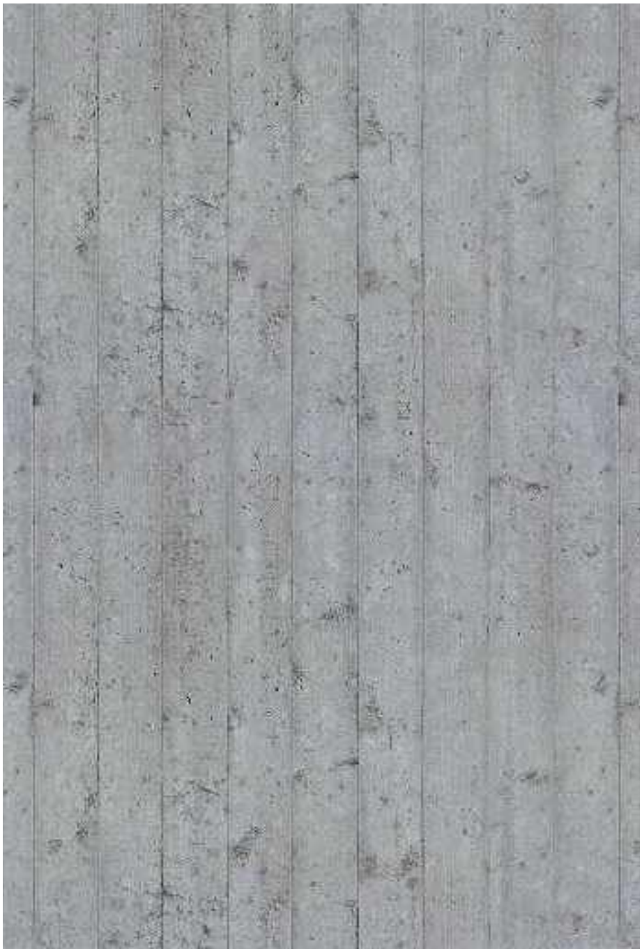
C. BOARD FORM CONCRETE ON STRUCTURAL AND BREAKAWAY WALLS
