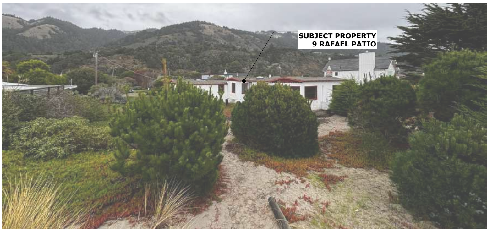
2 VIEW NORTH OF SUBJECT PROPERTY
