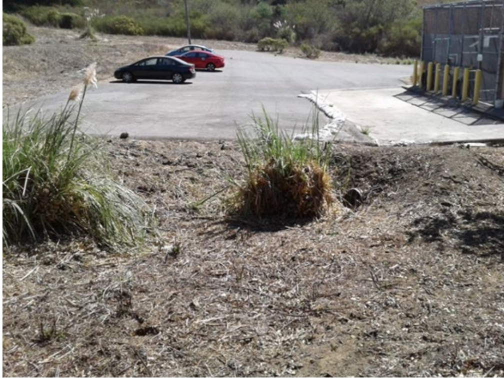
Photograph 12: Culvert at bottom of Drainage Segment 5-1.
