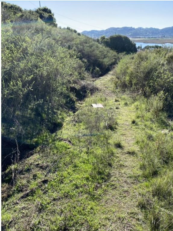
Photograph 6: Constructed diversion ditch (drainage segment 1-4) along access road (left side of photograph). Photo facing southwest.
