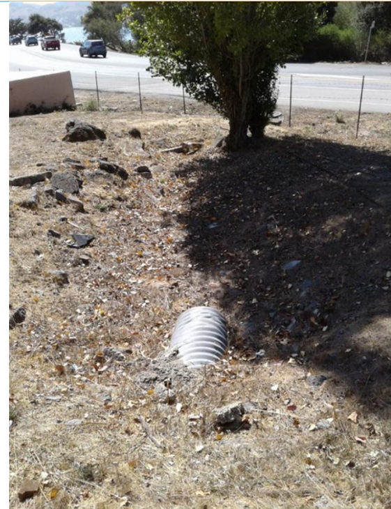
Photograph 11: Culvert draining into Segment 5-3 facing south towards Sir Francis Drake Boulevard
