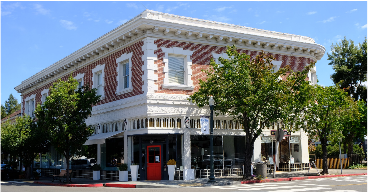
Example of Main Street Building
