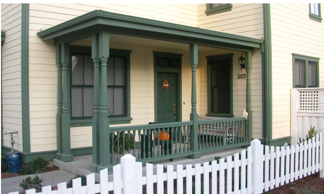
Example of an Engaged Porch
