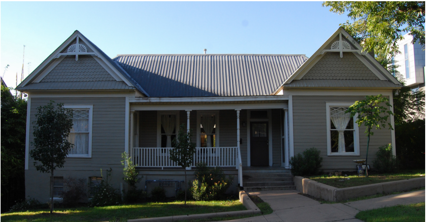
Example of an Engaged Porch
