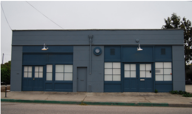
Example of a Maker Shopfront
