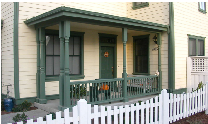
Example of an Engaged Porch
