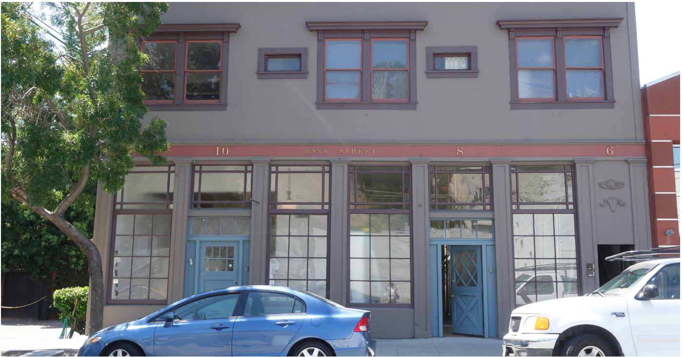
Example of a Maker Shopfront
