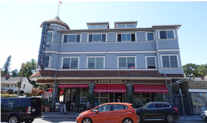
Example of Main Street Building
