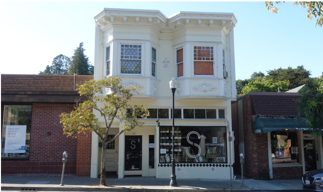
Example of Main Street Building
