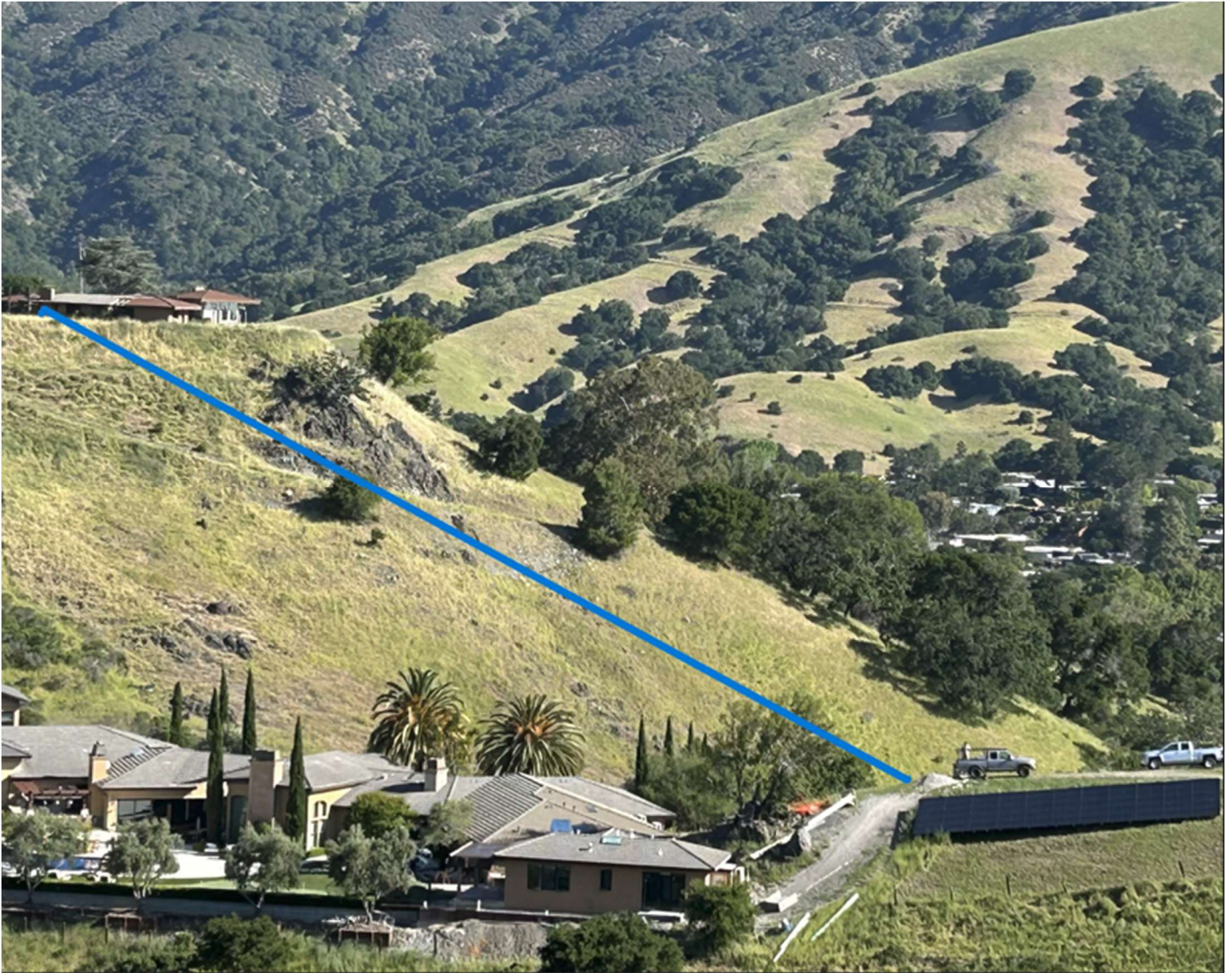
Photo 5 – taken from the Terra Linda fire road and depicting slope of hillside subject to developers proposed grading and drainage plans, and trees that will be removed, with Mike Stone’s residence in the foreground, and the existing home to be demolished in the left background. The line roughly depicts a 2:1 slope and the trees to be removed are depicted beyond the drawn line.
