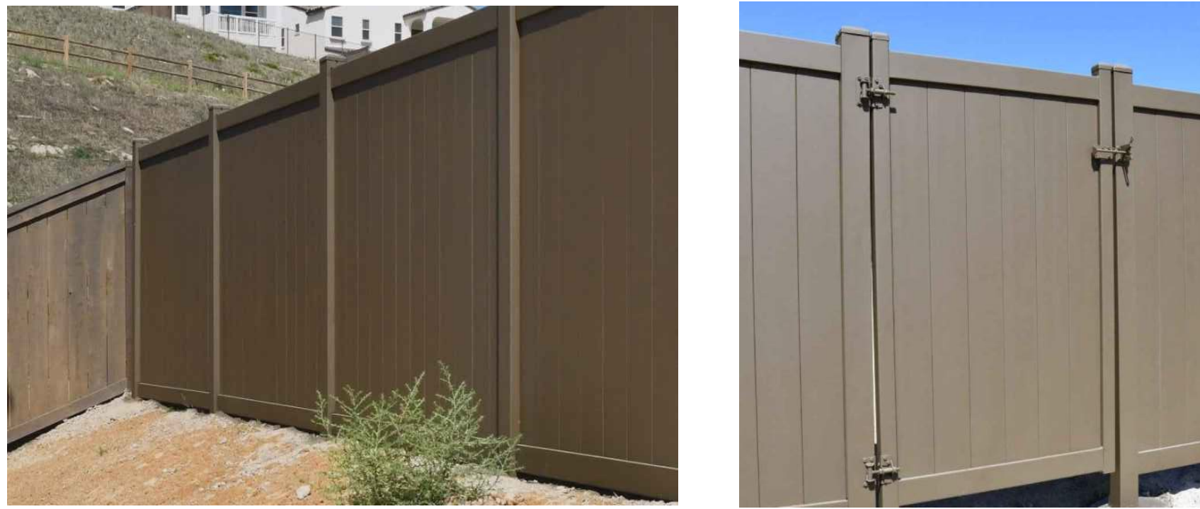
STEEL FENCE AND GATE SHALL BE: HAYDEN VERTICAL WITH 4" POST, COLOR: BROWN. AVAILABLE THROUGH MFW PRIVACY SOLUTIONS OR APPROVED EQUAL.
