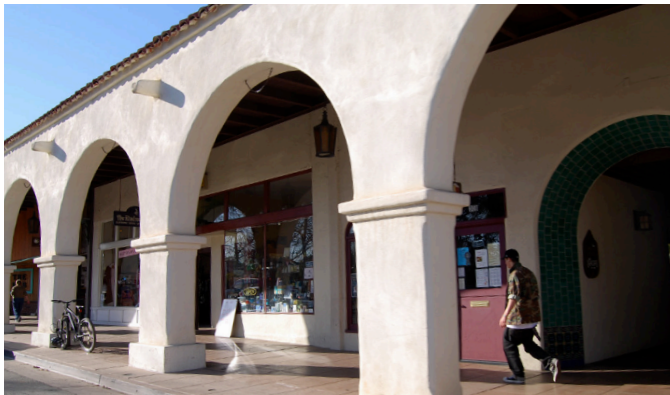
Example of a Gallery with shopfronts
