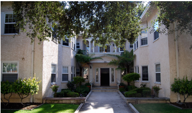
Example of Forecourt
