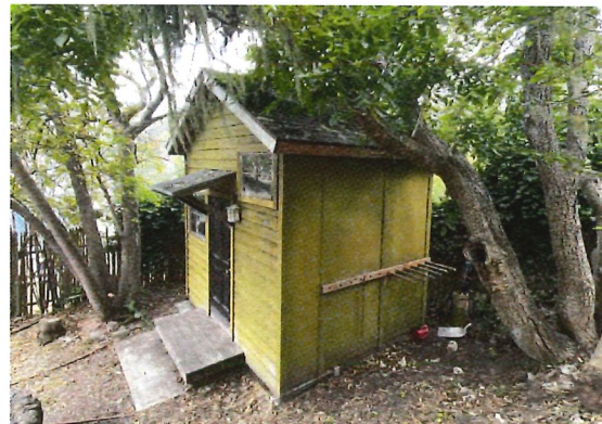
6 SHED EAST/SIDE ELEVATION
