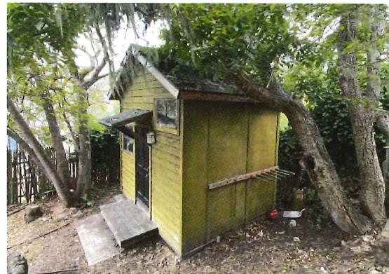
6 SHED EAST/SIDE ELEVATION
