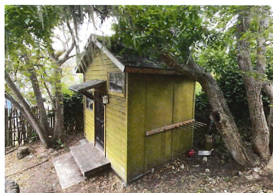
6 SHED EAST/SIDE ELEVATION
