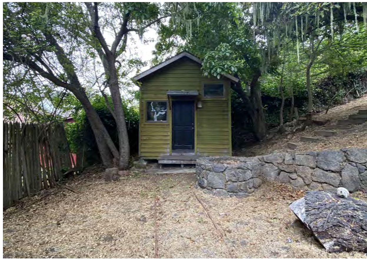
7 SHED SOUTH/FRONT ELEVATION
