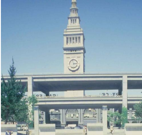
Figure 08. Ferry Building before removal of highway. Source: Ferry Building Marketplace Official Site.
