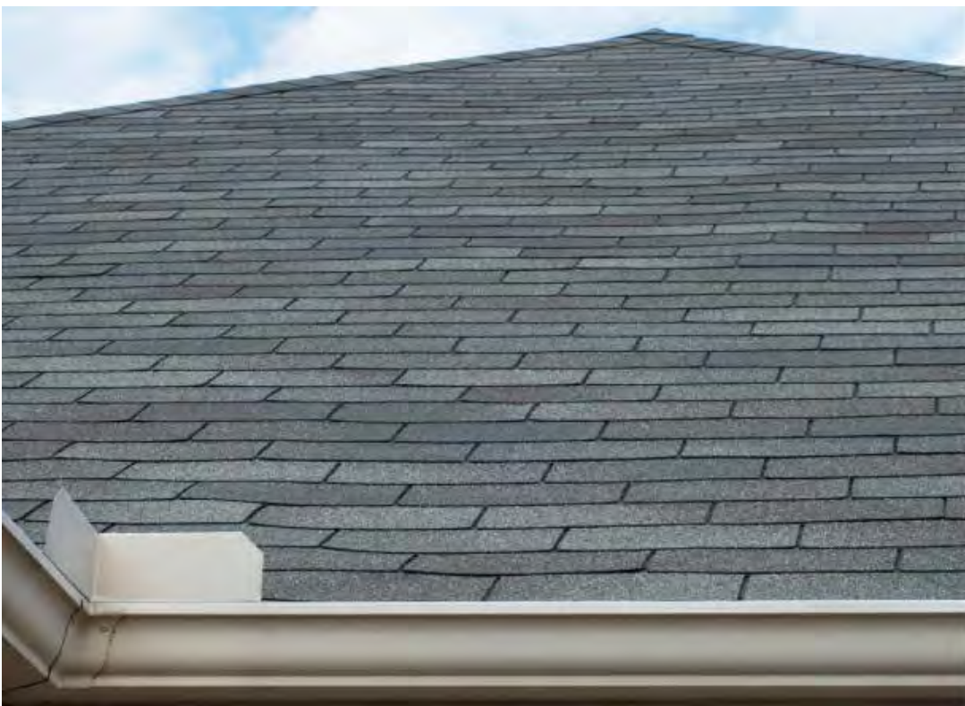
COMPOSITE BLACK SHINGLE ROOF
