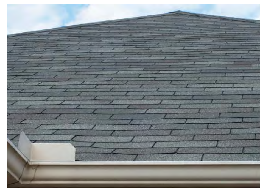
COMPOSITE BLACK SHINGLE ROOF
