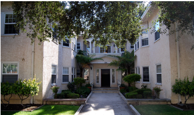
Example of Forecourt
