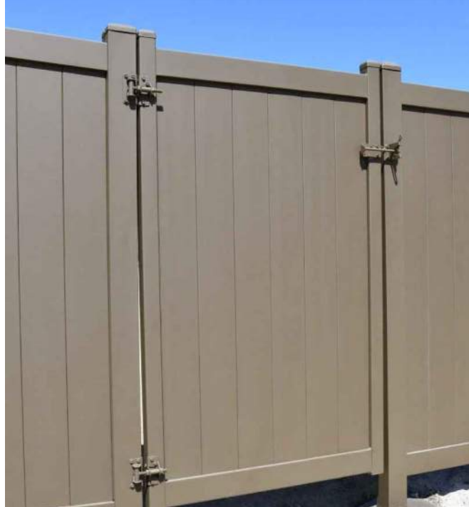
STEEL FENCE AND GATE SHALL BE: HAYDEN VERTICAL WITH 4" POST, COLOR: BROWN. AVAILABLE THROUGH MFW PRIVACY SOLUTIONS OR APPROVED EQUAL.
