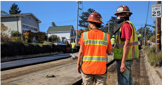
Department of Public Works engineering staff constructing and repairing road seals
