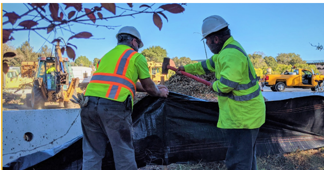
The Department of Public Works Roads Division preparing work at the Civic Center
