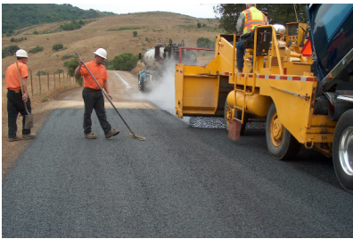
Public Works crews apply enzyme chip seal during road maintenance.
