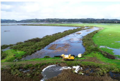
Flood control work underway at Simmons Slough.
