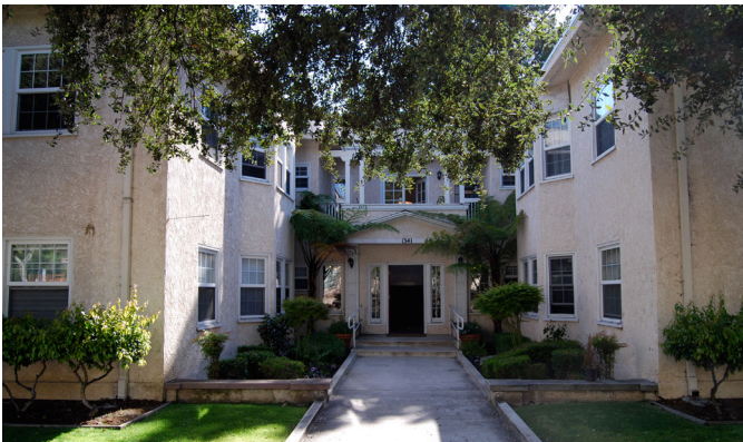
Example of Forecourt
