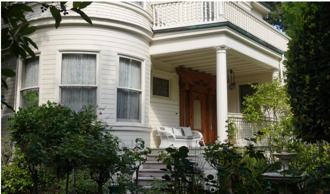
Example of a Projecting Porch
