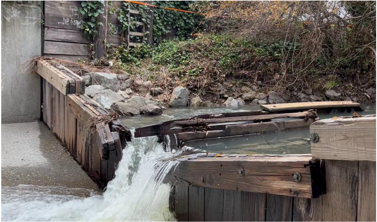
Figure 3 – Wooden Denil Fish Ladder, January 6, 2022
