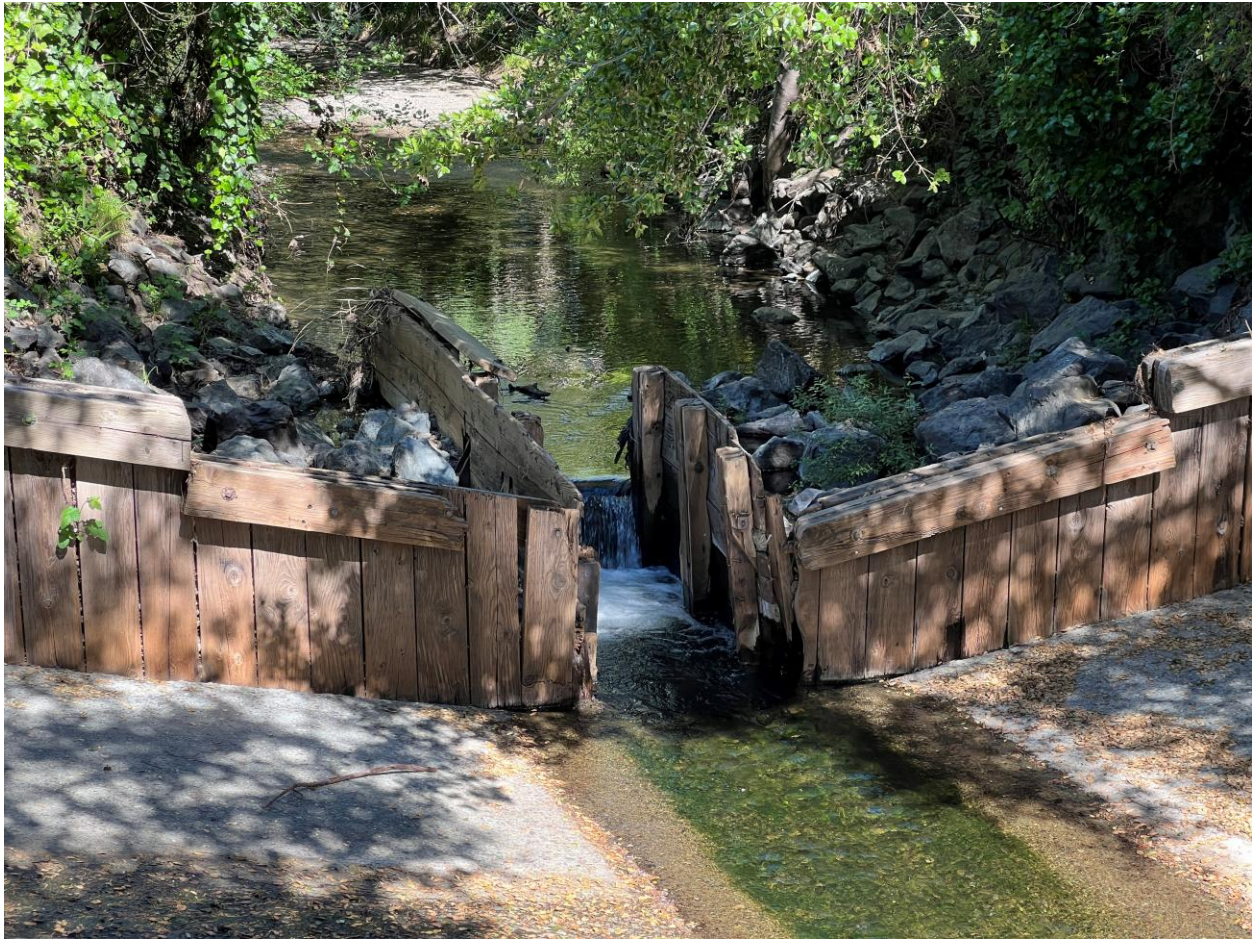
Figure 2 – Wooden Denil Fish Ladder, March 24, 2026
