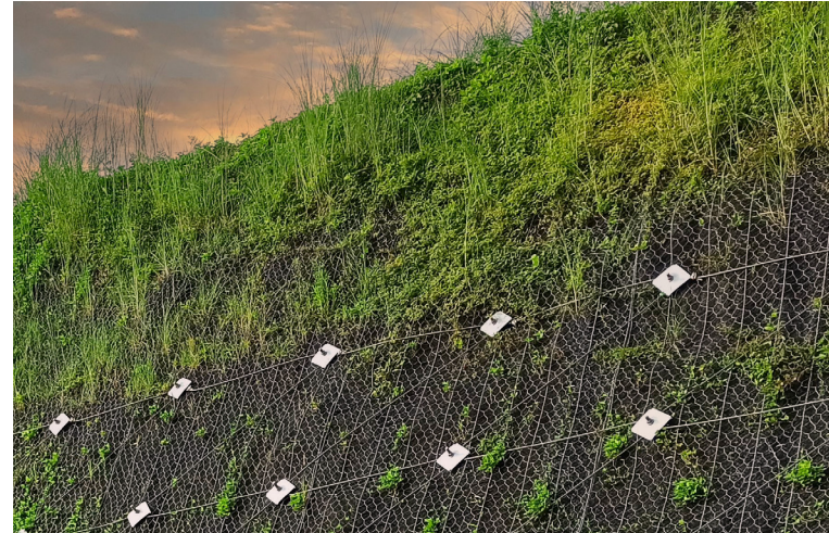
Soil Nail Wall with Vegetation.
