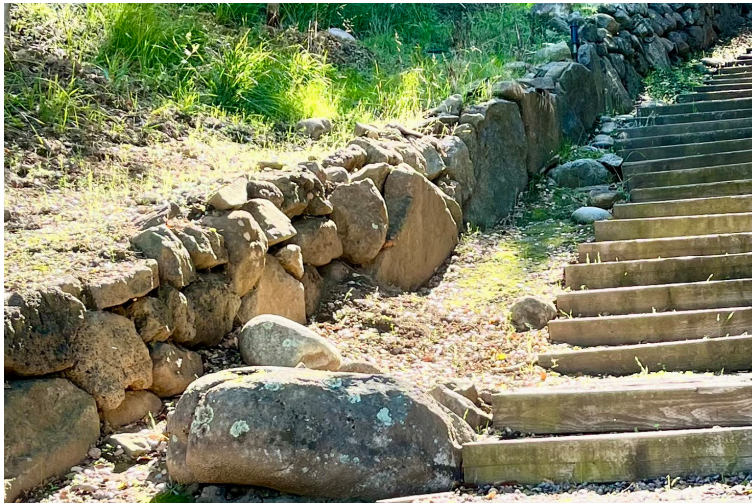
Timber tie steps at the Existing Fernwood Cemetery
