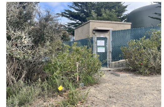
Existing Generator Shed
