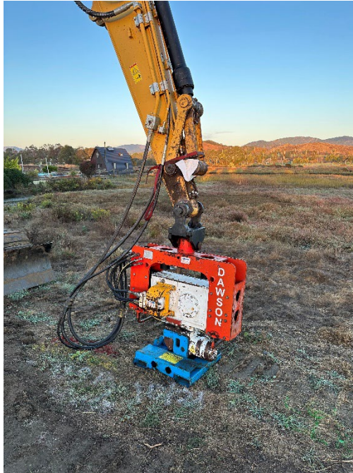
Photo 1: Vibratory hammer mounted on the end of an excavator used to install sheet piles.
