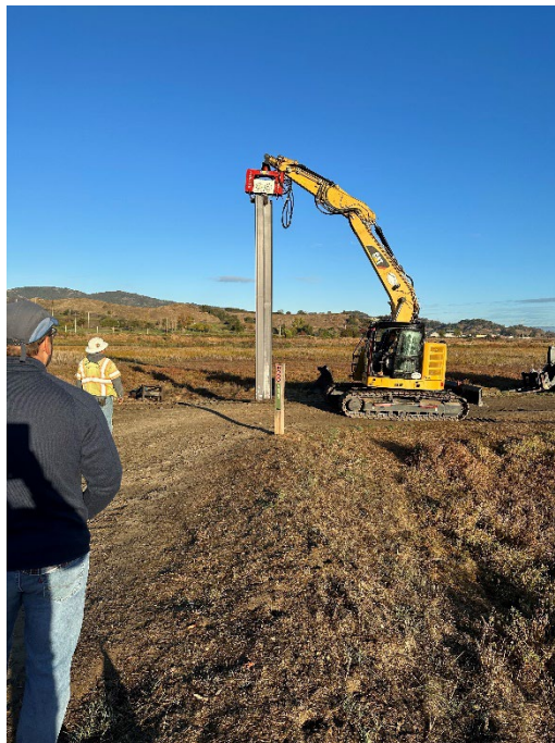
Photo 2: Excavator preparing to install a 20' sheet pile.
