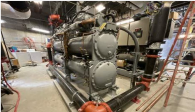
Mechanical system upgrades
