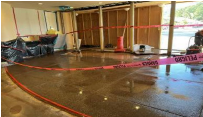
Lobby concrete slab replacement
