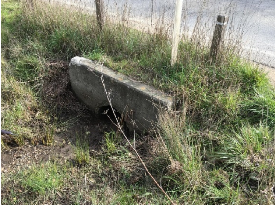
Photo 4. Degraded Culvert
