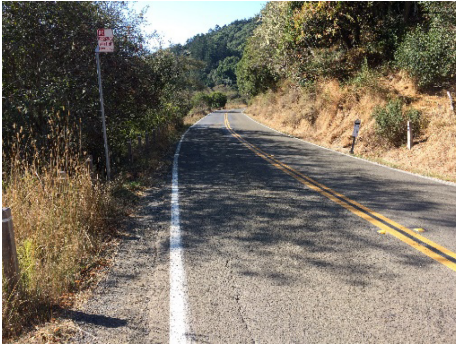
Photo 2. Narrow Road Width
