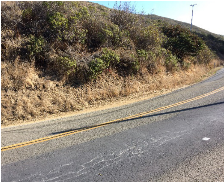
Photo 1. Pavement Deterioration
