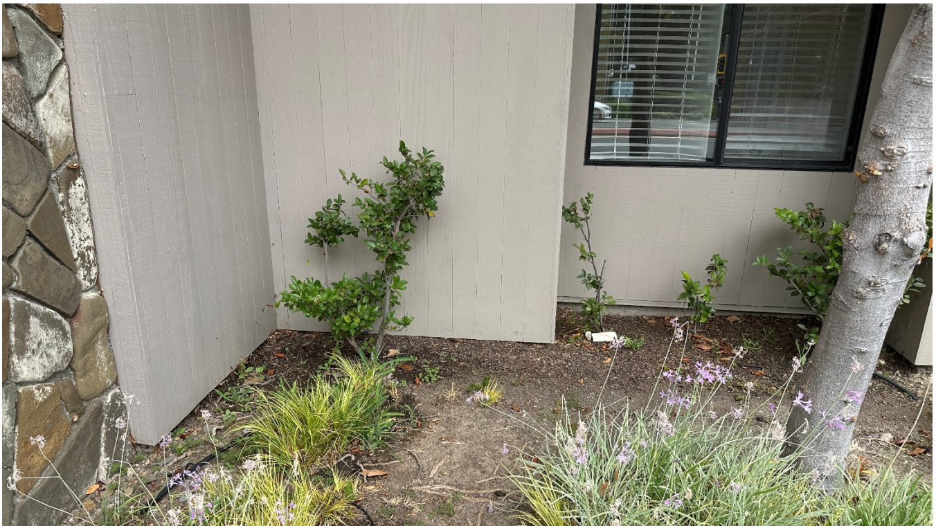
Photo 4: Grade at Building Perimeter
