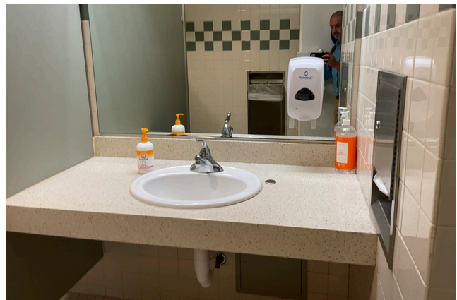
Existing Level 2 Public Restroom Lavatory
