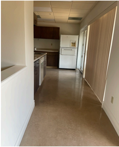
Existing Ramp to Level 3 Kitchen Area
