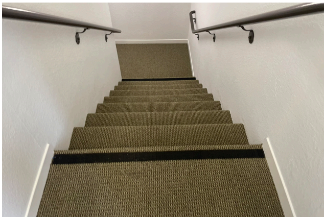
Existing Egress Stairs
