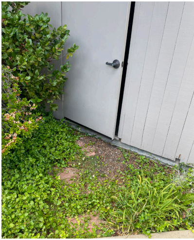
Existing Electrical and Telecom Closet
