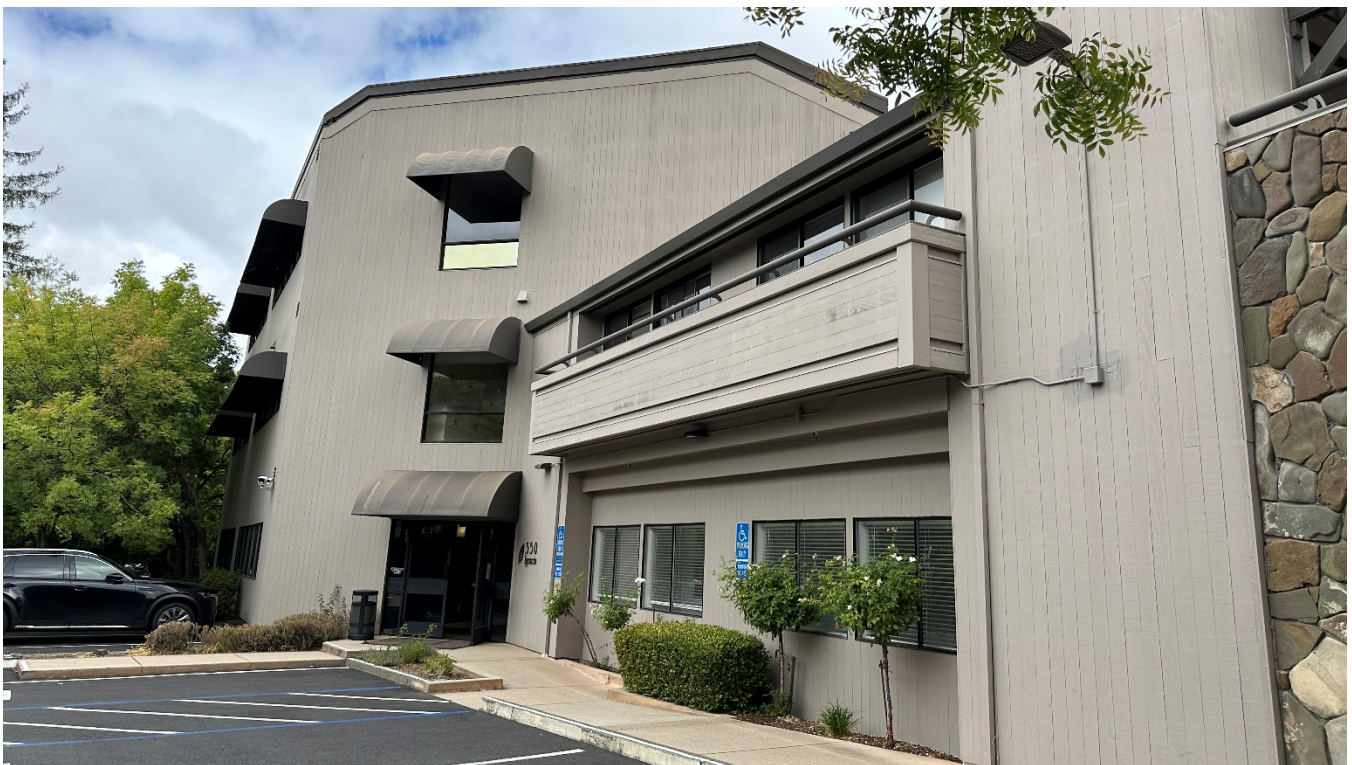
Photo 2: Building 1 – Southwest Corner
