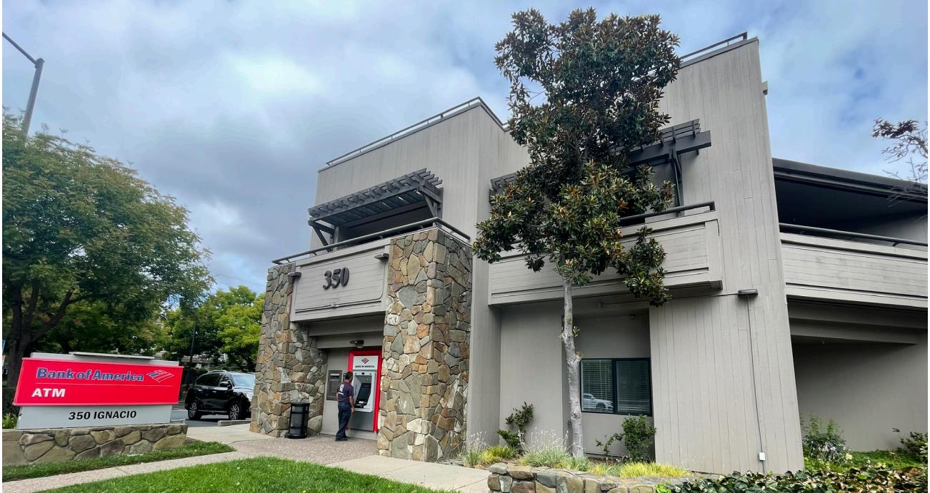
Three story, multi-tenant office building - South Facade
