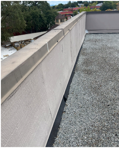
Exterior Roof Parapet
