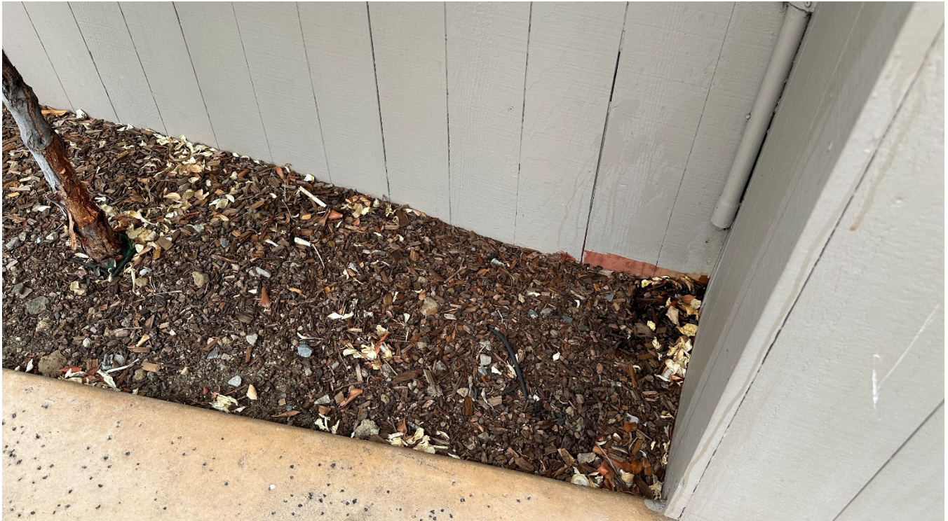
Photo 3: Grade at Building Perimeter
