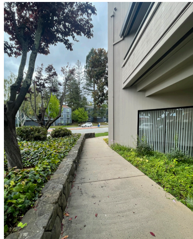
Perimeter Concrete Walkway around Building
