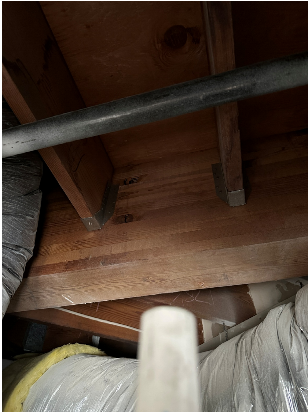
Photo 6: Structural framing above Mechanical Unit (First Floor)
