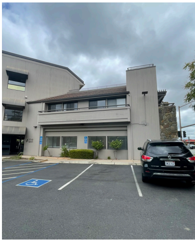
Existing ADA parking at Building Southwest
