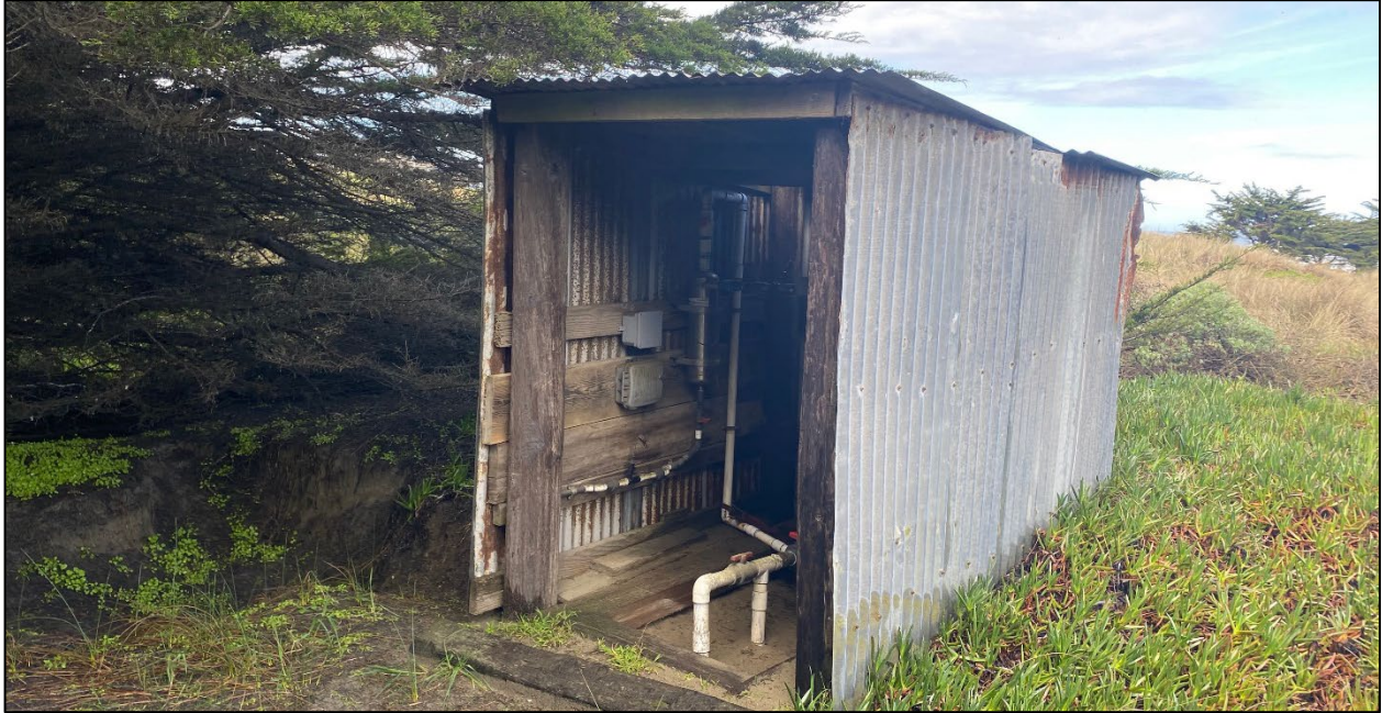
Photo 1. Existing, operational well.
