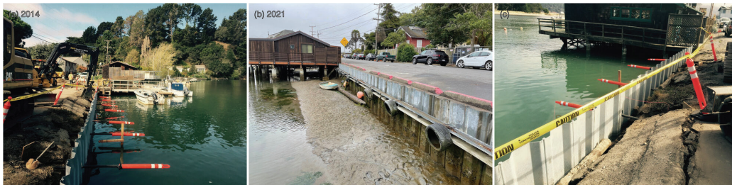
Figure 5 — Bolinas (Wharf Road) steel sheet pile seawall, designed by the author for the County of Marin: (a) installation, October 2014; (b) in service, August 2021 — no maintenance performed; (c) steel sheet detail October 2014
