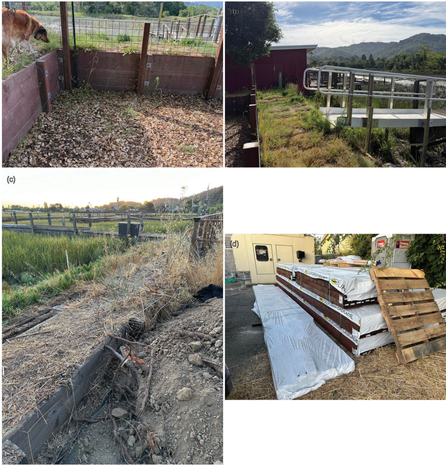
Figure 3 — Existing conditions along the TRB: (a) weathered timber wall at the rear-yard line; (b) gangway crossing the TRB to a private dock; (c) 2026 repair excavation along the timber wall; (d) repair lumber staged for berm patching. <mark>[Locations/dates to confirm.]</mark> Photographs: W. Tucker.
