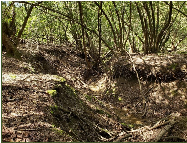
Head cut in drainage on southwestern side of the Bowman property.
